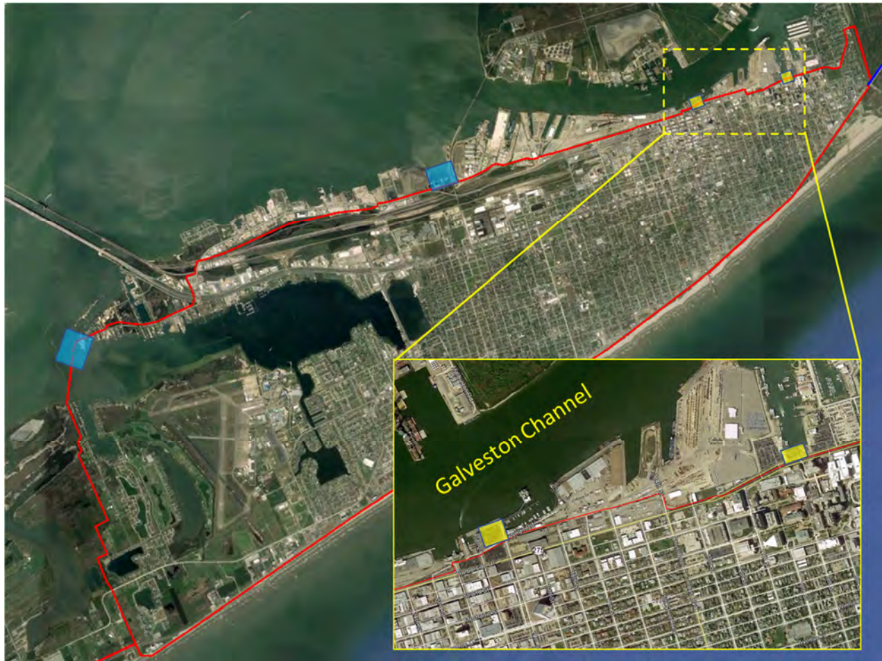
Figure 42. Aerial of the Phase 1 pump locations (blue rectangles) and the two new proposed pump sites (highlighted with yellow rectangles) at the northeastern side of the watershed; the Phase 2 analysis uses all four pump sites shown in this aerial.
