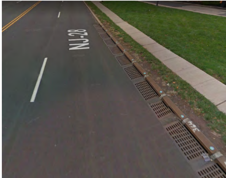
Figure 60. Google Maps Street View image of an example location with a set of inlets to capture extreme events along the road.
